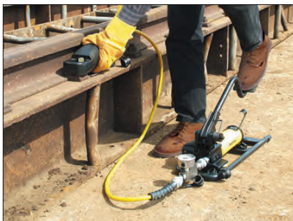
◀ Easily removing rusty nuts during railroad construction is just one of many application examples for the Enerpac Nut Cutters.
